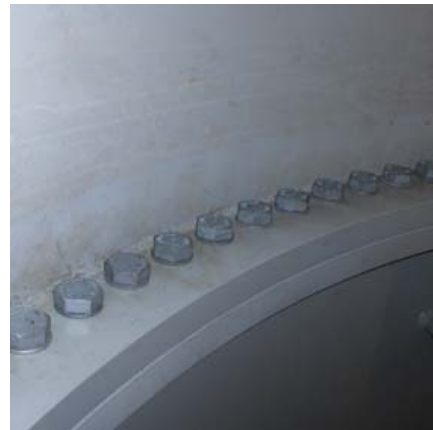
Internal flange connection
