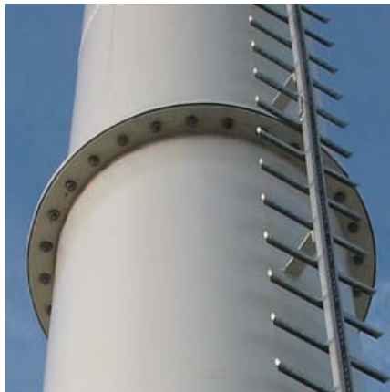
External flange connection
